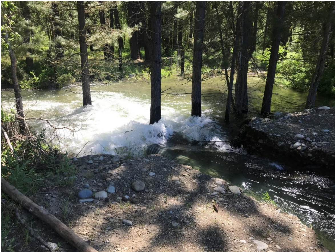
Figure 1. This photo was taken by Jennifer Nelson, WDFW, on June 6, 2022 from the edge of the pond immediately east of the Yakima River Campground property. This photo was taken from the adjacent property, looking at flooding toward the western portion of the Yakima River Campground property; near where the RV sites are proposed (electrical panel is visible between the trees, near center of photo).
